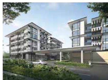
SINGAPORE THE VERANDAH RESIDENCES
